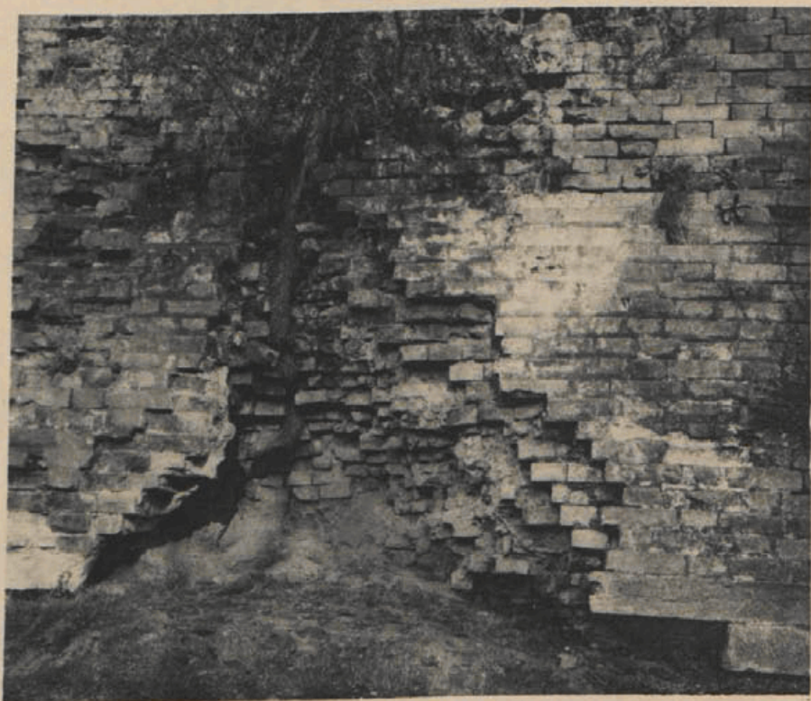
A deep hole in the east wall revealing several layers of the brick coating
