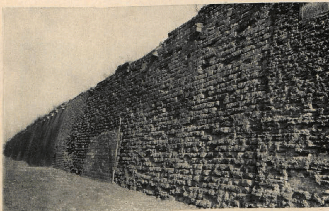
Badly patched and decayed portions of the inner east side of the Chinese city wall
