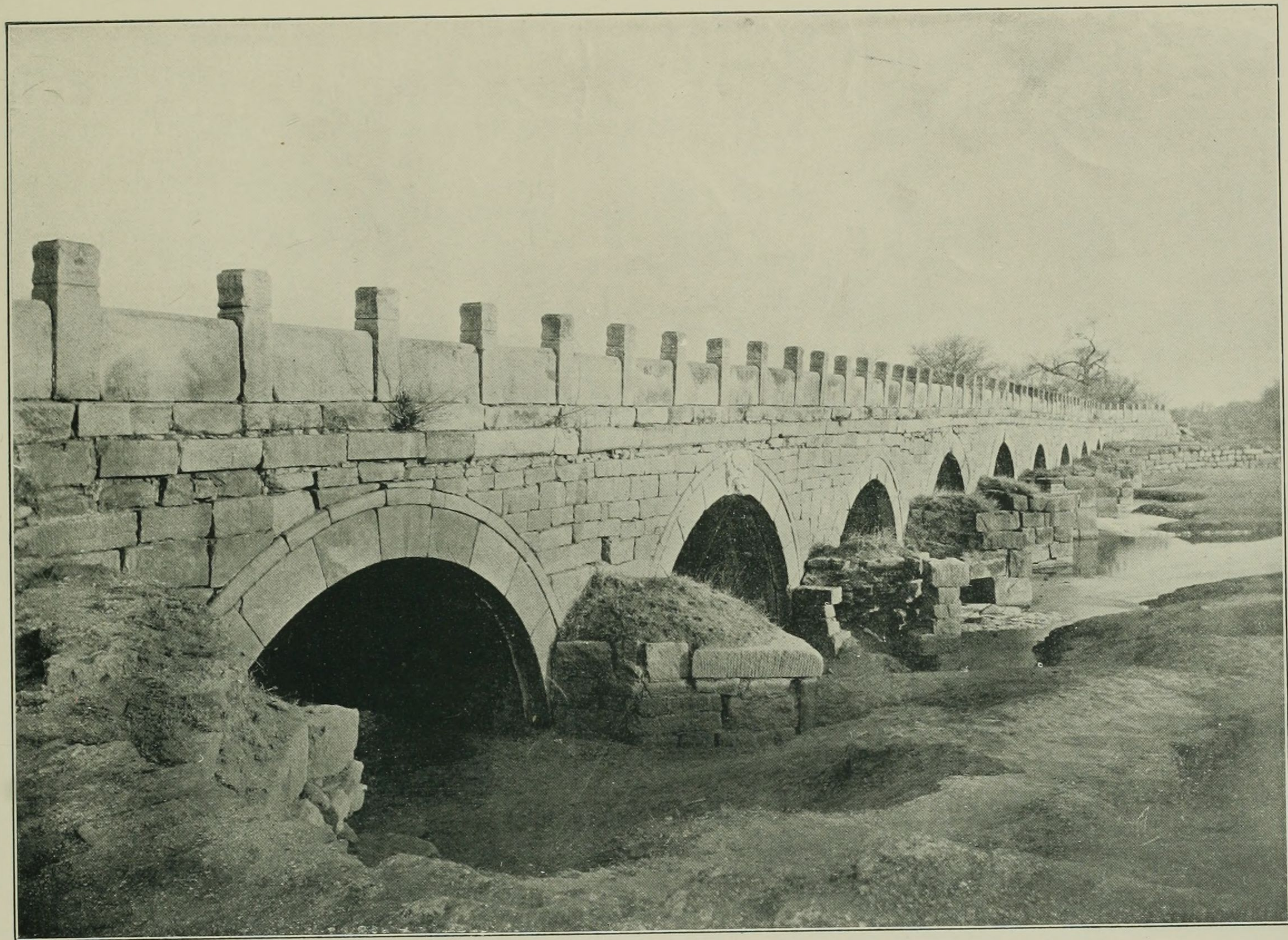
No. 61. Sha-Ho-ch'iao Bridge.
